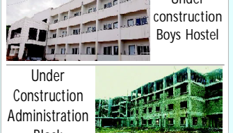
Under construction Boys Hostel
