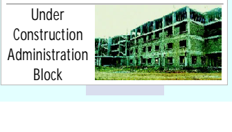
Under Construction Administration Block
